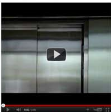
VIDEO: Leonard Florence Center modified the elevators to enable operation via remote control.
